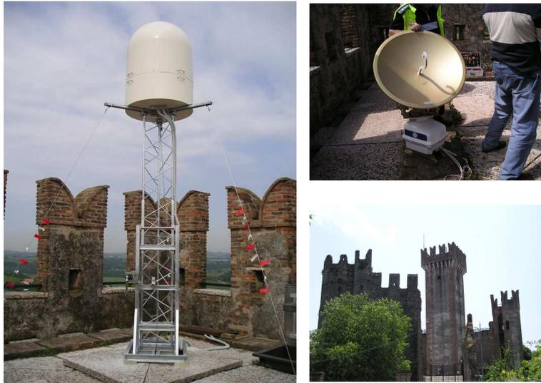
**Figure 3:** Left: X-band radar installed on the main tower of the medieval castle of Valeggio sul Mincio (Verona, Italy). Right: (high) the antenna of the radar and (low) view of the castle.
