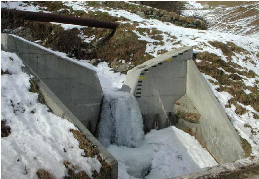
**Figure 1:** IFKIS Hydro observation site in the area of the Simplon Pass (Valais, Switzerland). During intensive rainfall periods, local observers pass at this site in regular intervals collecting information about water levels, bed load depositions and other important information.
