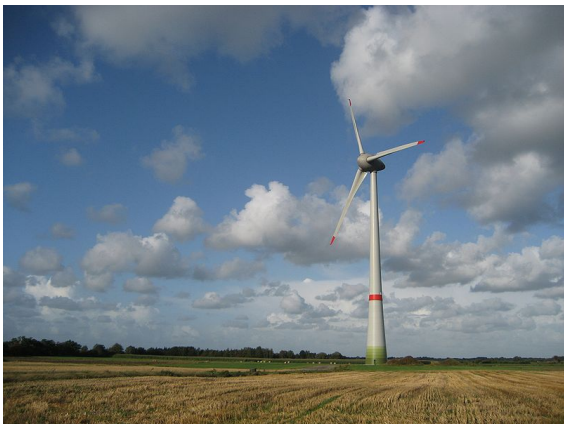
Figure: Enercon E-126 wind turbine: largest to date with hub height of 135m, rotor diameter of 126m and total height of 198m (Source: Wikipedia).
